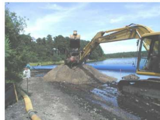
Iron filing barrier installation within the shoreline at Ashumet Pond, Falmouth
