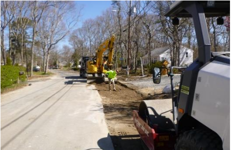
Construction: Temporary Paving
