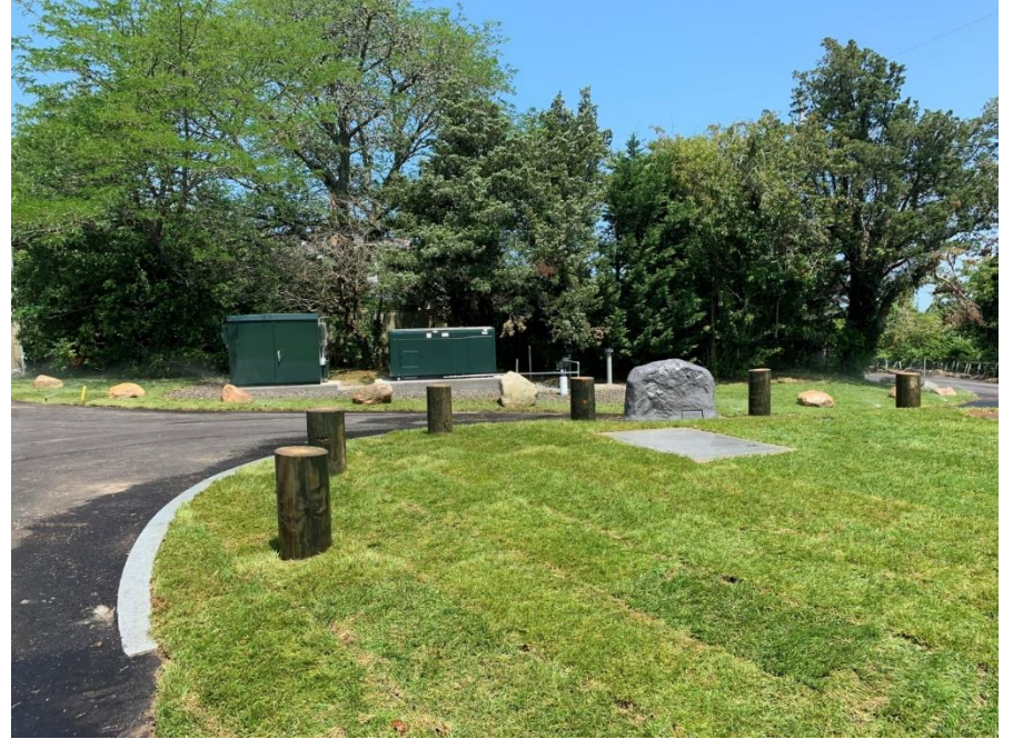
Rendezvous Lane Pump Station
