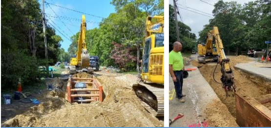
Construction: Excavation & Sewer Installation
