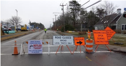
Construction: Road Closures / Detours
