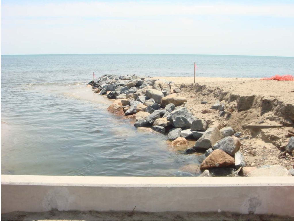
Figure 5-51: Rushy Marsh New Inlet, Newly Installed, Perspective Looking Toward Nantucket Sound
