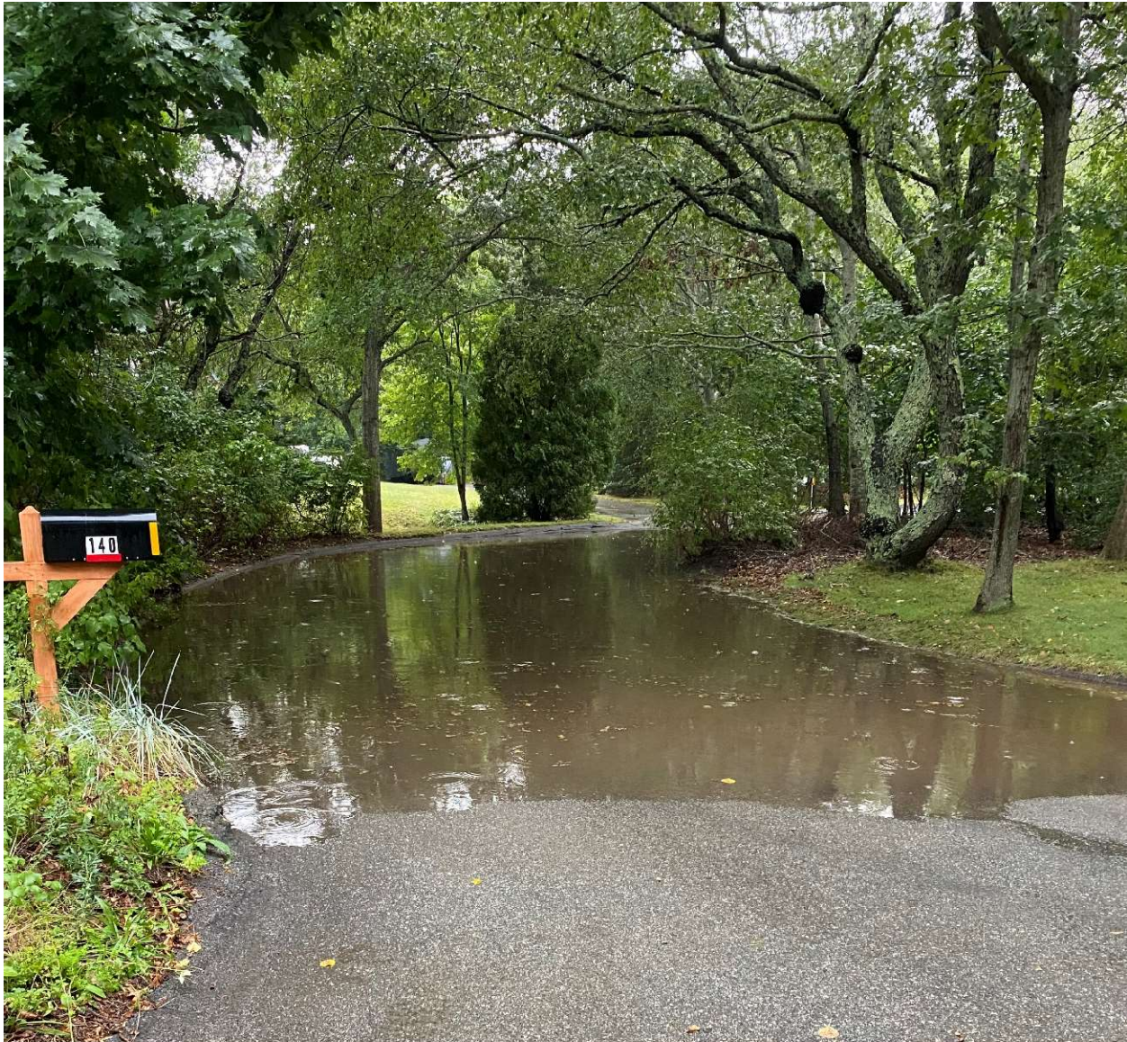
Figure IV-32. Stormwater ponding on Willimantic Drive. Willimantic Drive loops from Race Lane to Cotuit Road. At the turn toward Cotuit Road, Willimantic Drive becomes a private road and there are no catch basins in this area. Project staff identified a partially occluded pipe and headwall west of the boat ramp that may be connected to this area. This picture of ponding was taken after rain had stopped following the 9/28/21 storm.
